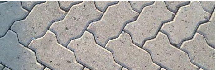
Driveway | Continuous footpath treatment
