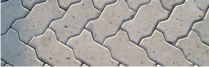
Driveway | Continuous footpath treatment
